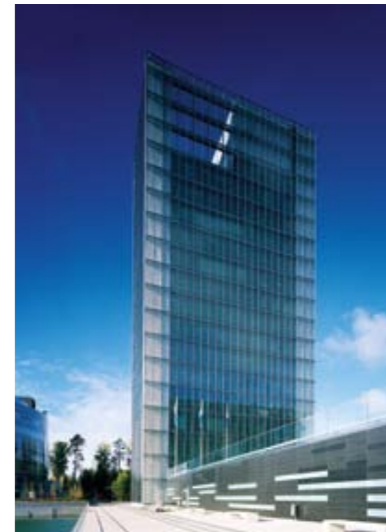
Multi-tenant office building • 16 floors, 4-car group Typical features: • Audible guidance for disabled • DOP's with dot matrix
