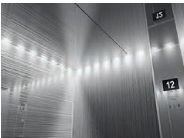
Actual CL181 ceiling installed in car
