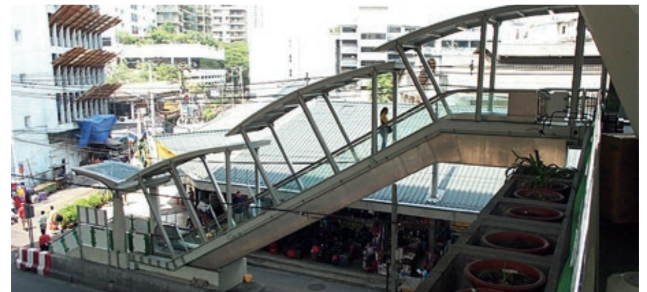
Figure 4.3 The outdoor escalator should be covered by a roof to improve passenger safety and convenience.
